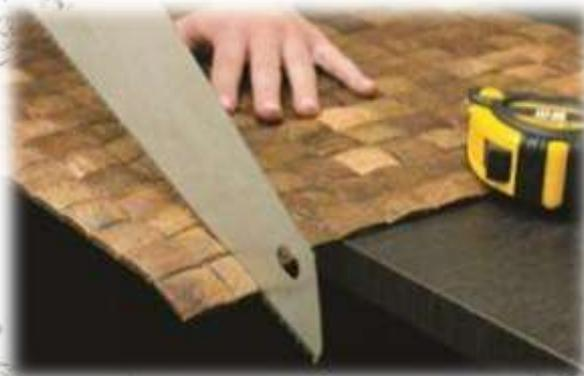
For cutting of mosaic not at the place of joint (along a coconut cell) use an angle grinder, electrical fret saw or an arm-saw.
