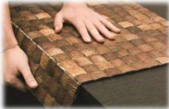
For cutting of mosaic at the place of joint break it along the joint on the edge of a table. Then cut a glue base with a sharp utility knife.
