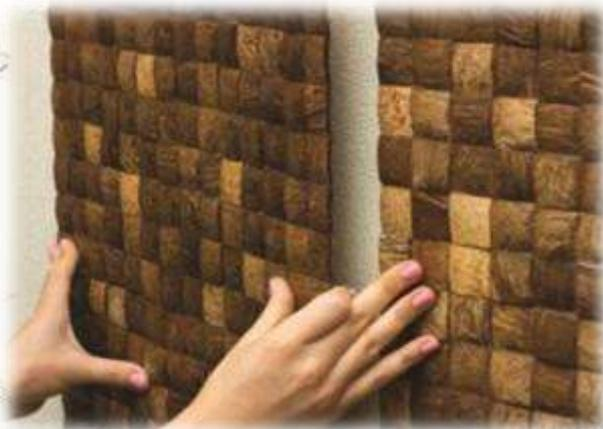
Press a panel with glue to the surface. It is necessary to press the panels marry in to each other.
