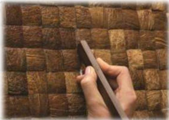
After drying up of the glue you need to use a wax crayon Cosca to hide the joints between panels.
